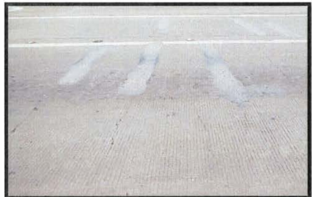
Concrete Spall Repair – Grand Parkway frontage road
