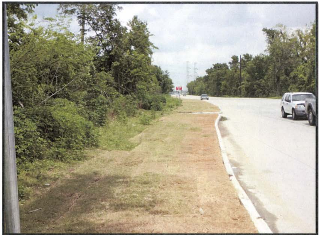
Sod placement – southbound frontage road
