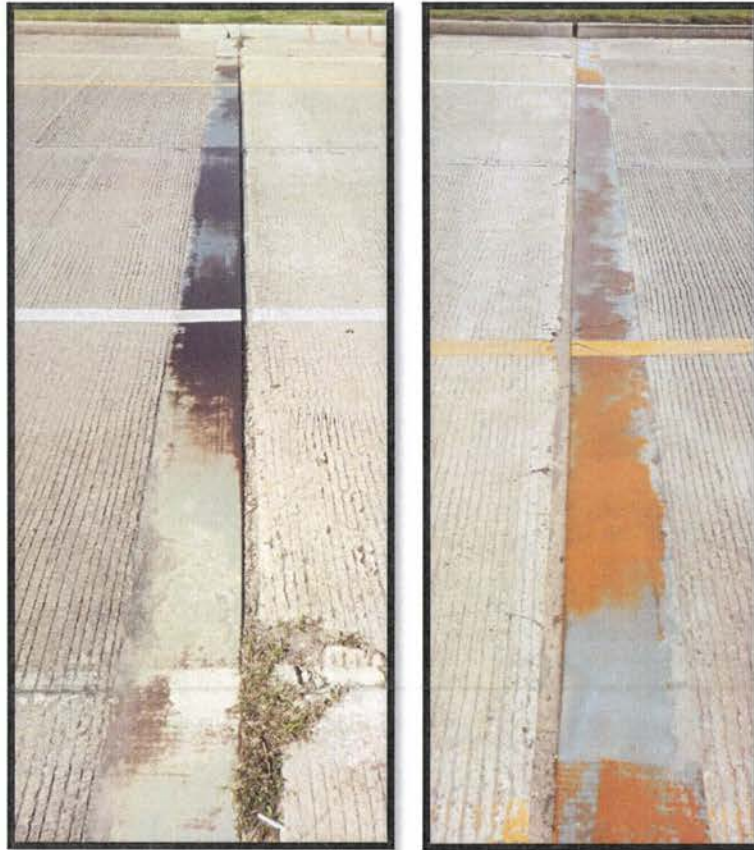
Before and after – replace expansion joint material
