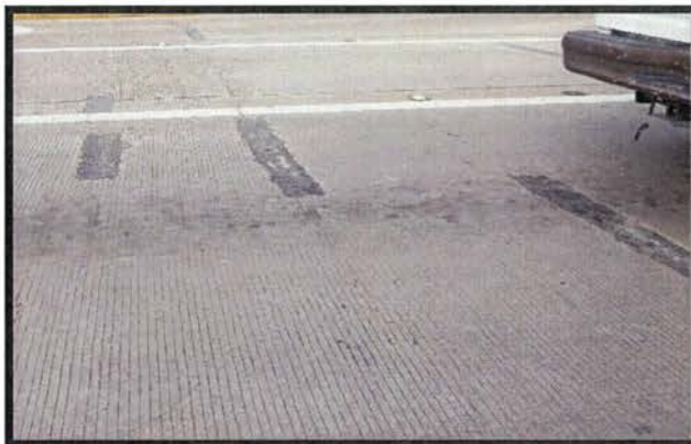
Concrete Spall Repair – Grand Parkway frontage road
